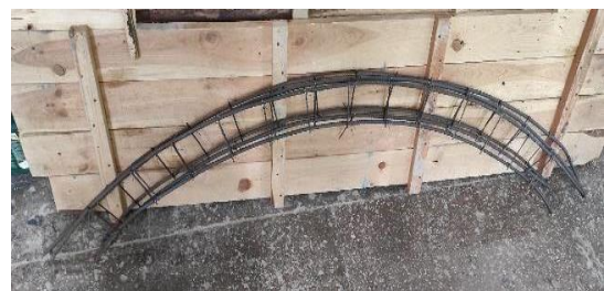
Fig. 2. General view of the manufactured frame.
