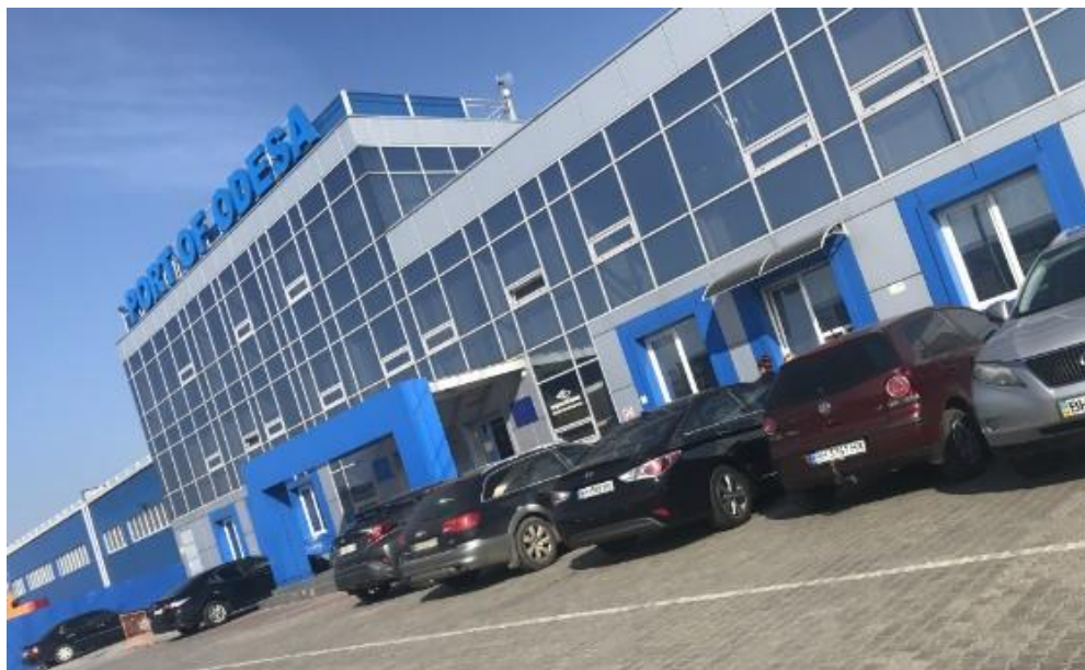
Fig. 1. General view of the building before the missile attack
