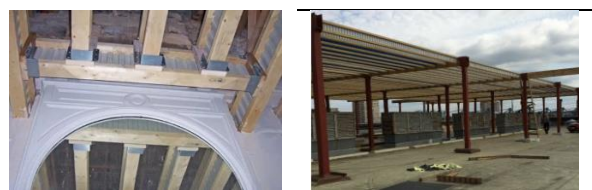
Fig. 9. The use of metal-timber beams during reconstruction
