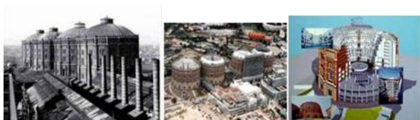
Fig. 1. Renovation of the gas holders in Vienna
