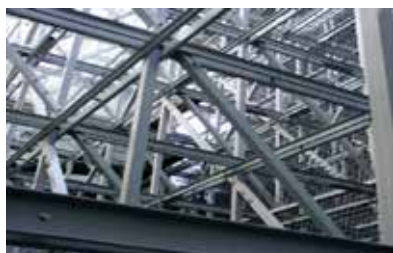
Fig.1. General view of the application of fiberglass structures
