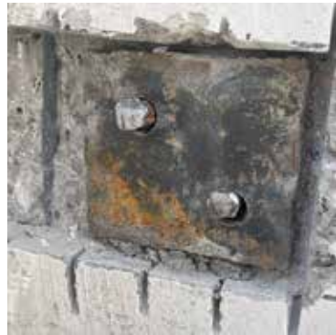
Fig. 2 - Prepared for welding insert on chemical anchors
