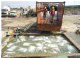
Fig. 2. Using ice to form a concrete mix.
