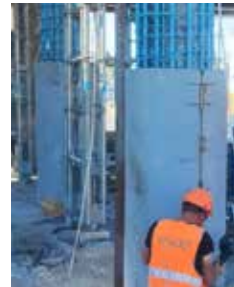
Fig. 2 – Installation of additional reinforcement and installation of fixed formwork shell
