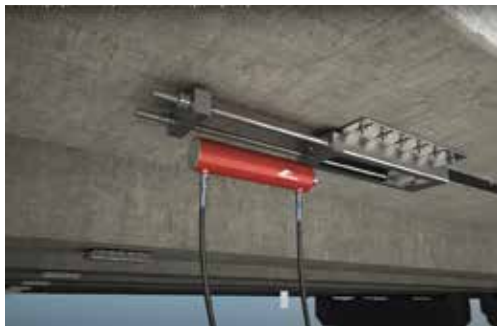
Fig. 2 – Installation of composite external reinforcement with external strengthening
