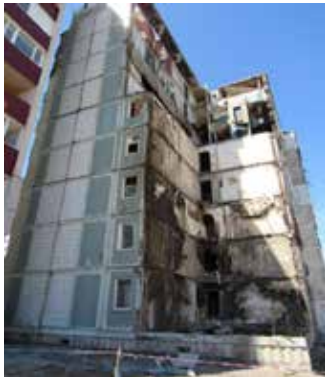
Fig. 1 - Destruction of part of the block section of a large-panel multi- apartment building at 25 Zakhisnyky Ukrainy St. in Uman
