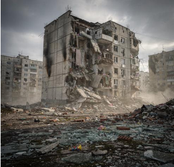
Fig. 3. Severe structural damage with partial collapse, Kharkiv (example of severe to destroyed classification)
